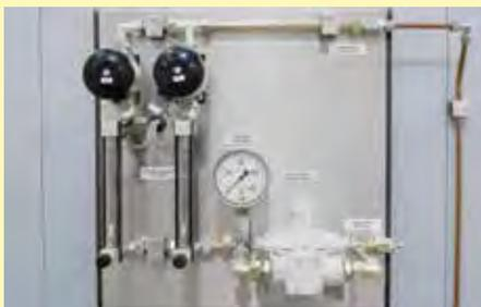
Gas supply system for non-flammable protective or reaction gases
