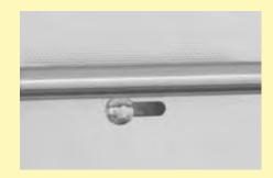
Adjustable air inlet integrated in the door
