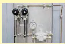
Gas supply system for non-flammable protective or reaction gases
